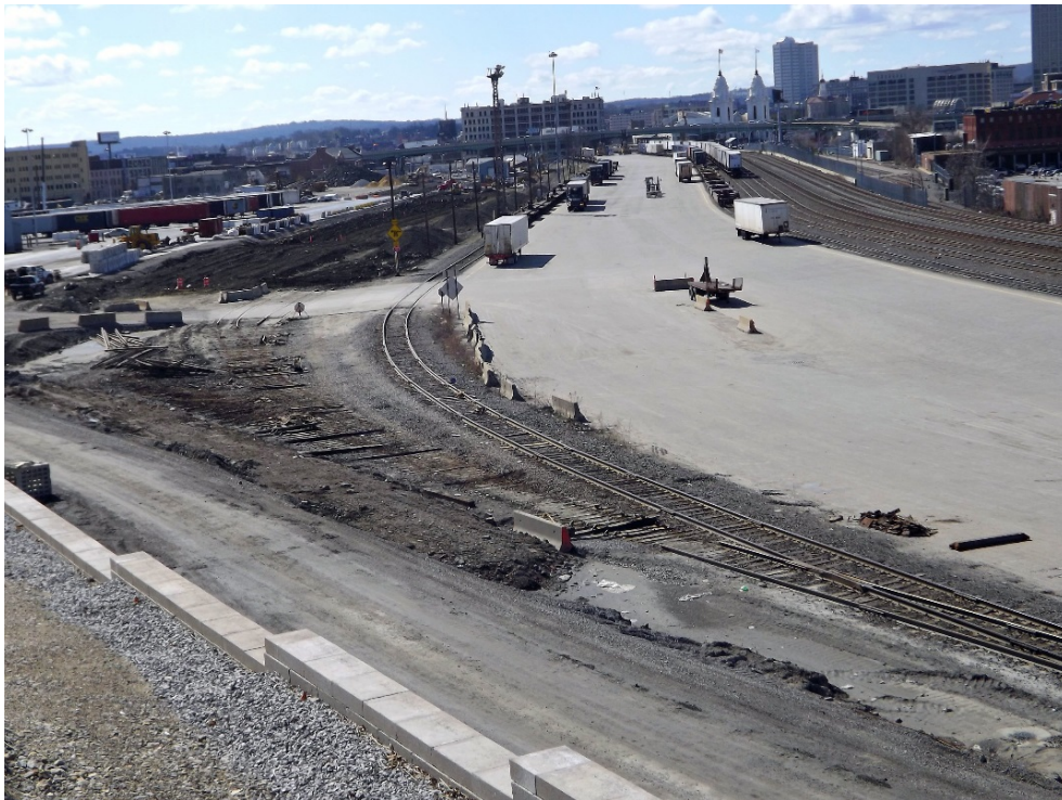
Expansion dirt work
