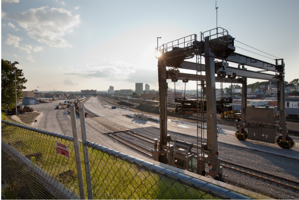
Railway expansion completed
