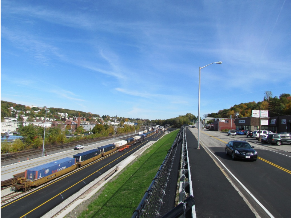
Roadway improvement above
